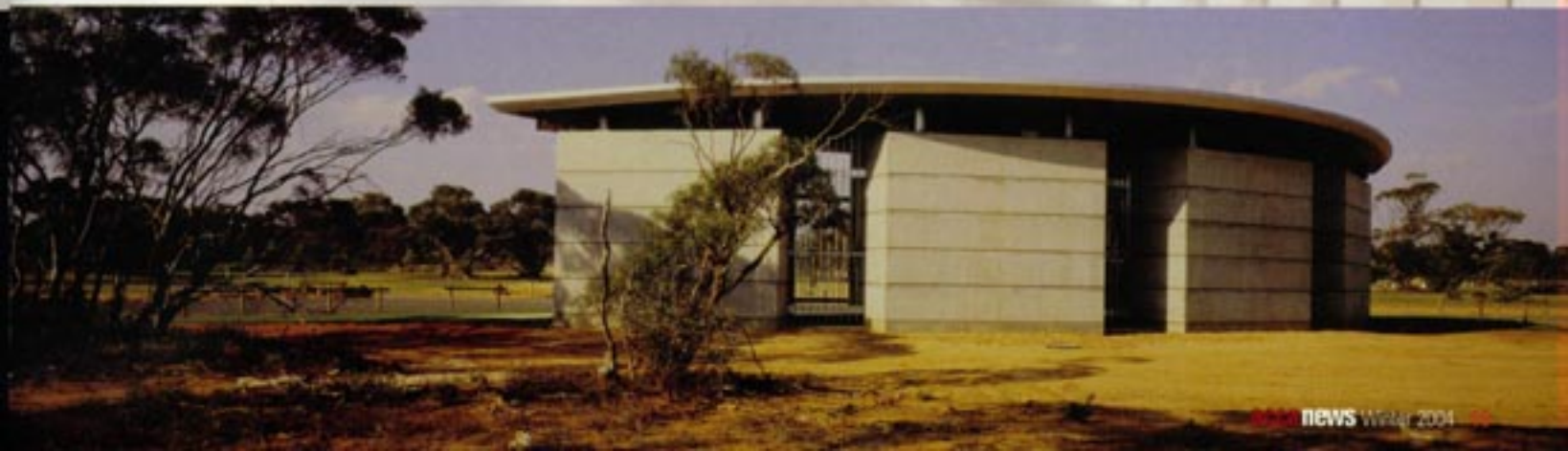
Below: Landscape conservation zone
