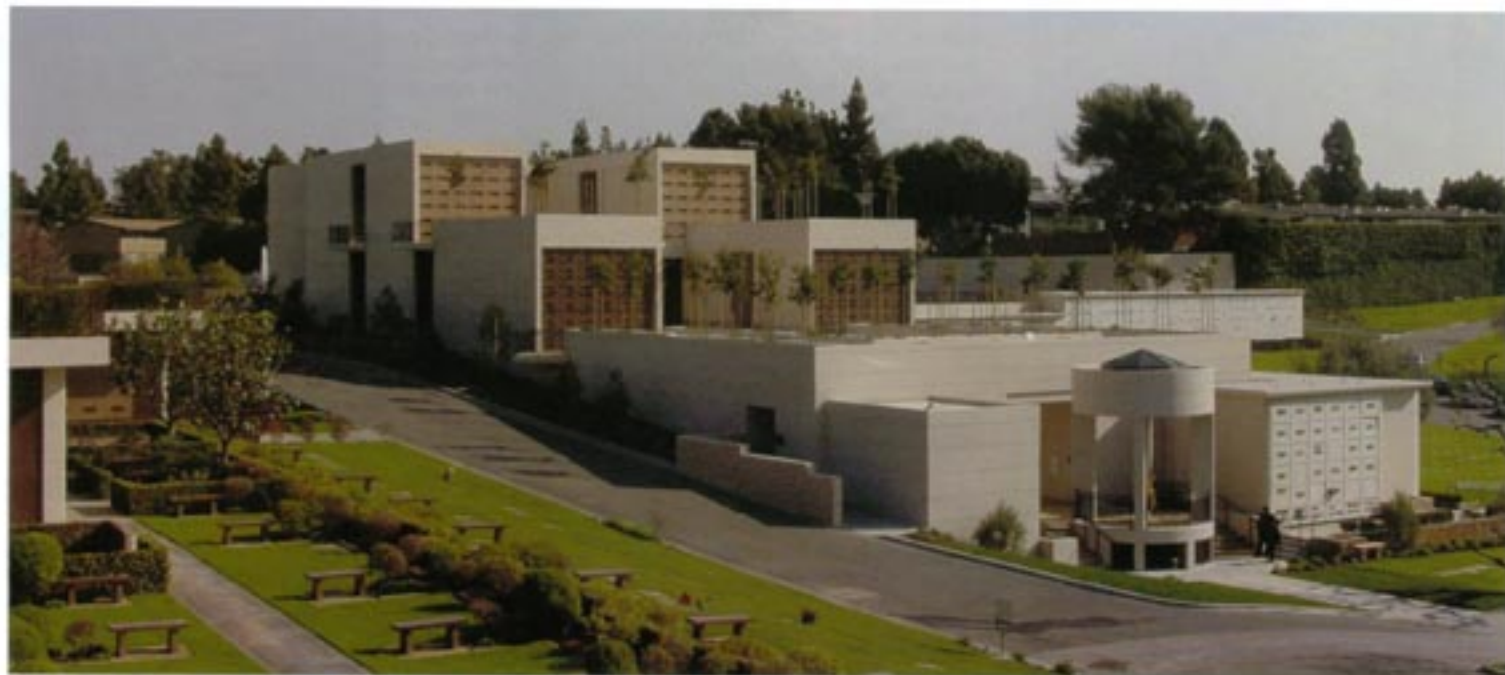
Hillside Memorial Park and Mortuary's new Court and Garden of the Matriarchs mausoleum and lawn crypt project takes up 40,000 square feet of a 2.6-acre site. The three-level mausoleum and the lawn gardens (see photos on pages 32-33), which are terraced, were designed to fit on a difficult site, basically a ravine. The project also was designed to be "neighborhood friendly," and to complement the existing buildings in the cemetery. At far right in the photo, to the right of the pavilion, is part of Sunland Gardens, an L-shaped garden mausoleum already present on the site and integrated into the plans for the new building. To the left is the Canaan garden crypt complex.
